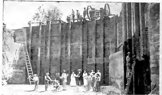
FIG. 3.—ENTRANCE GATES IN FRONT, FLUSH AND WASTE GATES AT RIGHT.
